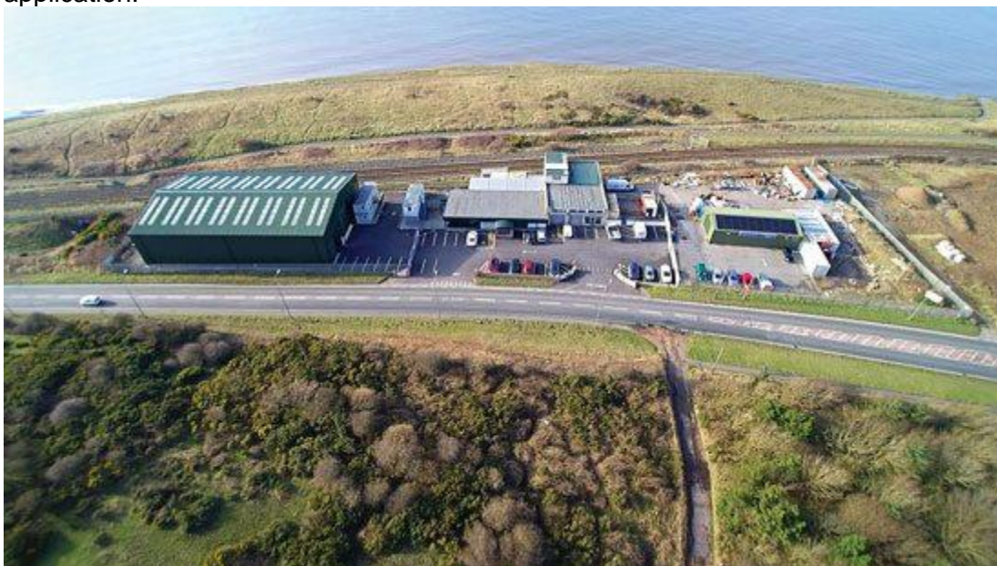
The EM&I Technology Centre at Forth Engineering in Cumbria.
