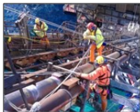
Piping / Vessel R&M
