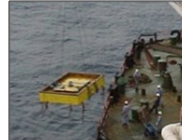
In-Water Structural R&M
