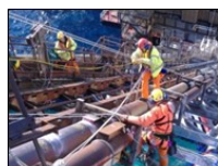
Piping / Vessel R&M
