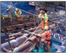
Piping / Vessel R&M
