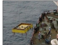
In-Water Structural R&M
