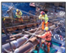
Piping / Vessel R&M
