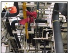
Lifting Gear Inspection
