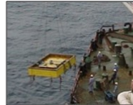
In-Water Structural R&M
