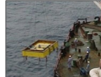
In-Water Structural R&M
