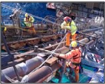
Piping / Vessel R&M
