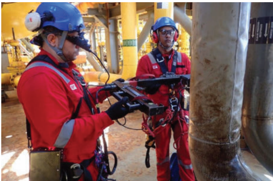
Real-time radiography screening of corrosion under insulation.
