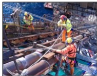
Piping / Vessel R&M
