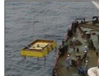
In-Water Structural R&M
