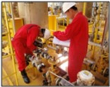
Pressure System Inspection
