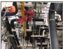
Lifting Gear Inspection
