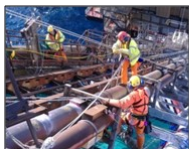
Piping / Vessel R&M
