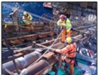
Piping / Vessel R&M
