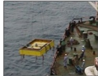
In-Water Structural R&M
