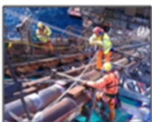
Piping / Vessel R&M
